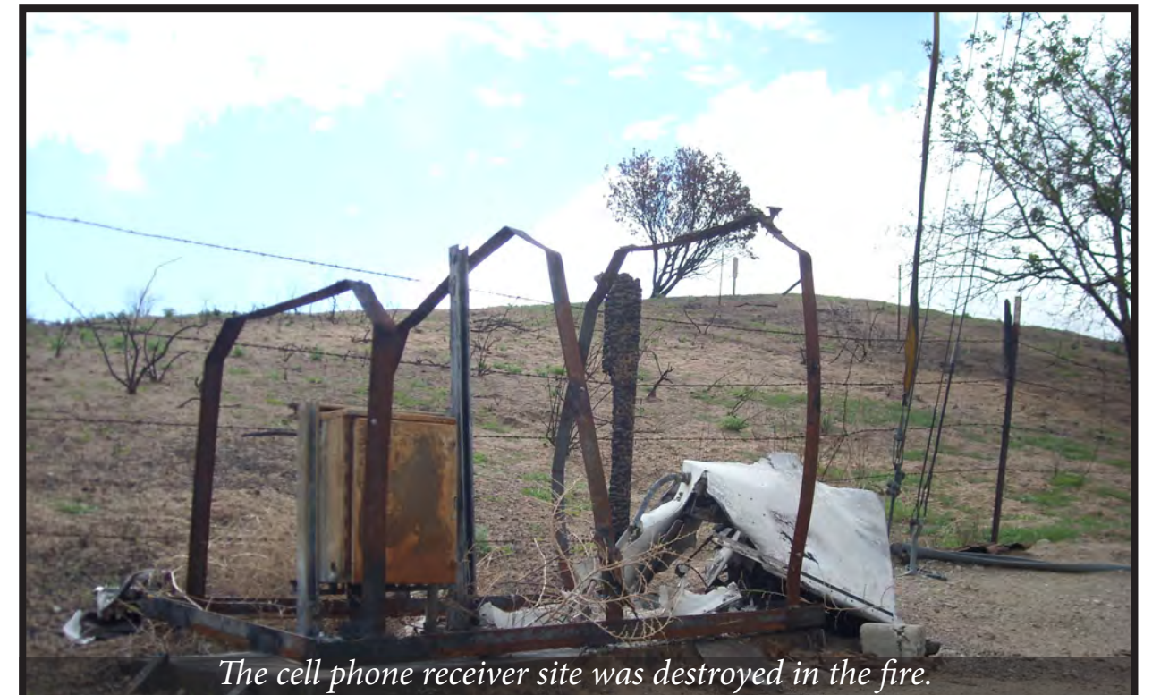
The cell phone receiver site was destroyed in the fire.
