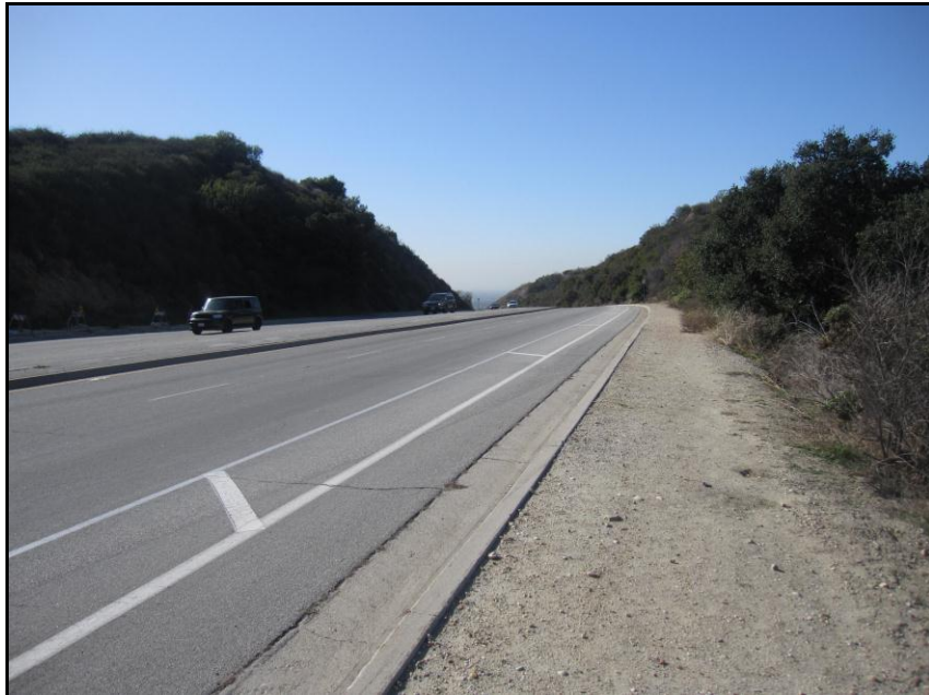
Figure 3. Cut slopes along Colima Road.
