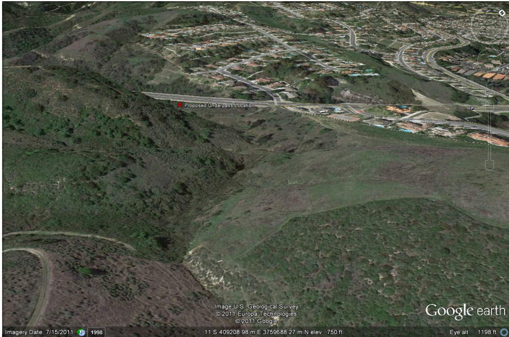
Figure 8. Looking west along upper Arroyo Pescadero at the proposed underpass location, east portal.
