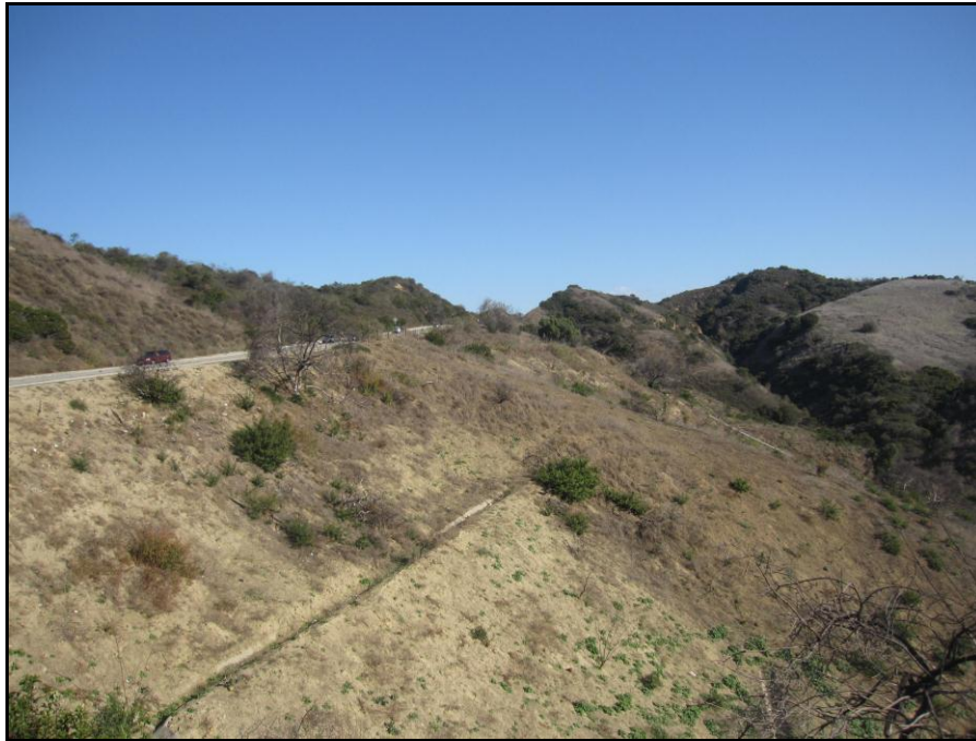
Figure 2. Example of a fill slope (fill slope 4).
