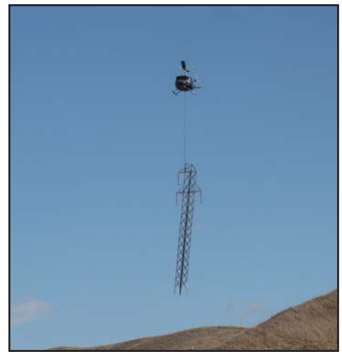
Obsolete tower being carted off by helicopter.
