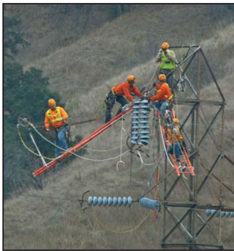
Edison crew at work disassembling the tower.
